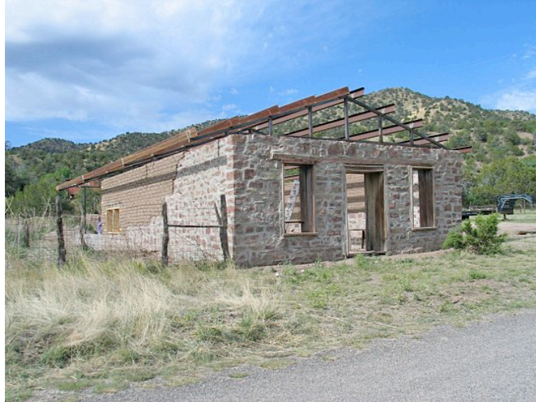
Restoration of old bank building, Chloride.
